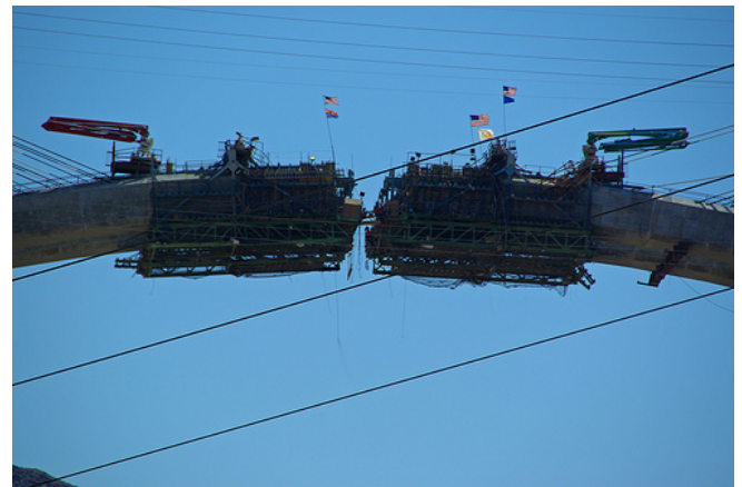
Arch inching toward completion
